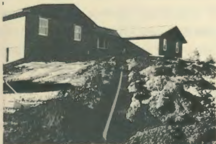
Special drainage was a requirement.
