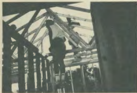
Tom, working high in the ceiling joists.....
